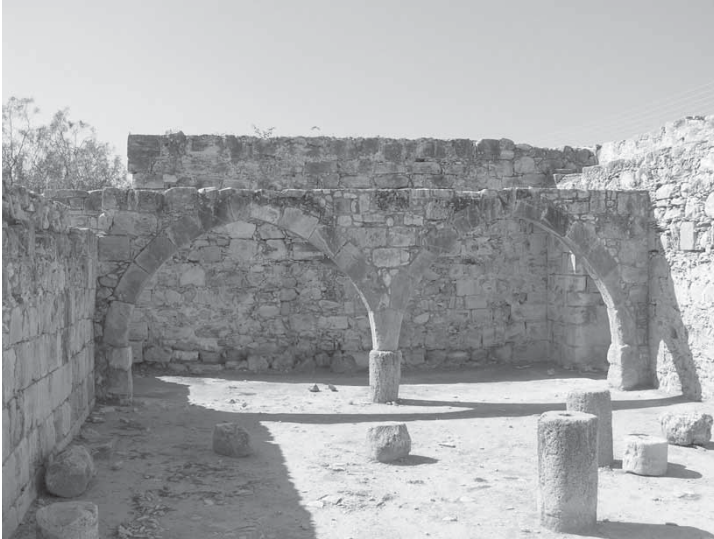
Fig. 79: Kolossi, two-storeyed rectangular building to the southwest of the keep, view of the ground storey towards the south [M. Olympios].
